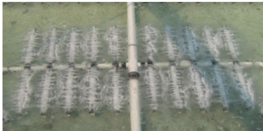
Tubular fine bubble diffusers were installed during this Retrofit that also included replacement air header, drop pipes and blowers.
