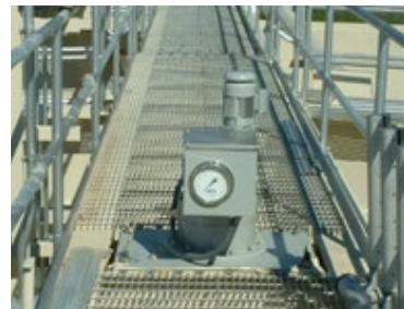
New Clarifier Drives
