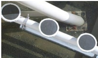
Close-up view of a circular fine bubble diffuser recently installed on a retrofit project.
