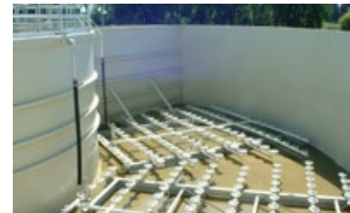
Replacement circular fine bubble diffusers were installed during this retrofit project.
