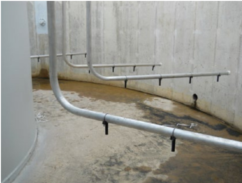
New stainless steel drop pipes, stainless steel drop pipe assemblies and MULTIFUSER™ diffusers were installed at this Illinois treatment plant during this retrofit project.
